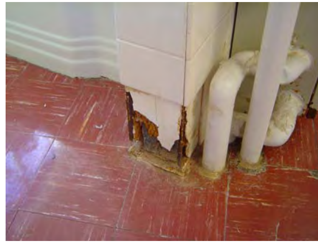
Deteriorated plaster and metal stud wall.
