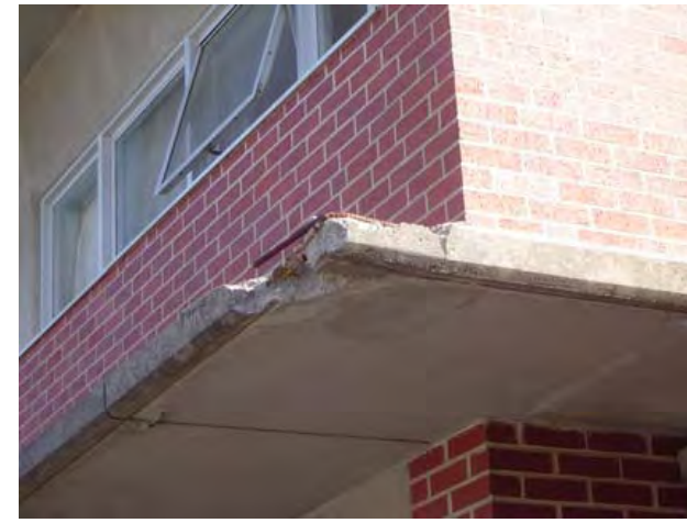
Damaged concrete shading eyebrow.
