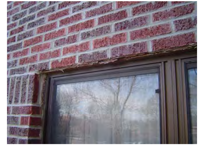
Deteriorated steel lintel above windows.
