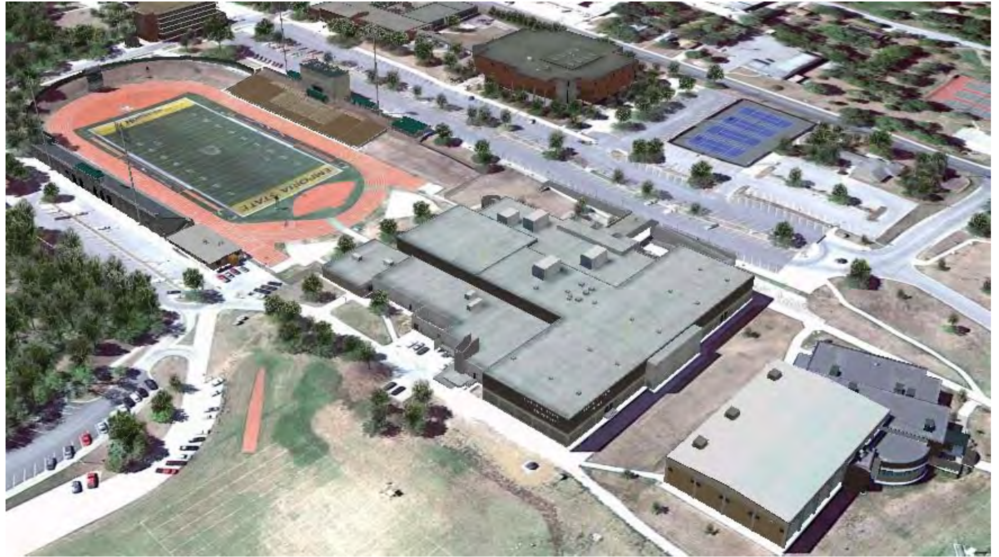
Welch Stadium, Health / Physical Education / Recreation Building, Student Recreation Center
